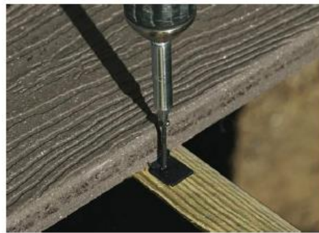
Hidden Fastener Installation to Joist
